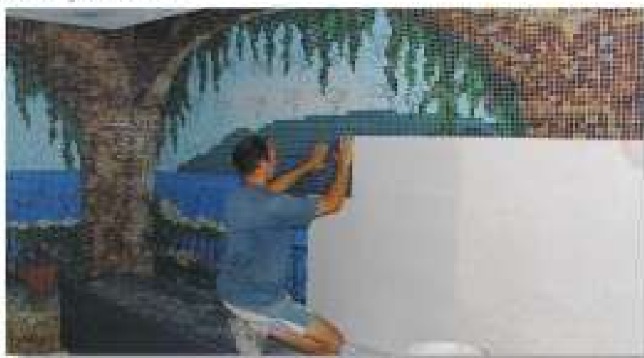
Burkolás. Assembly to the wall.
